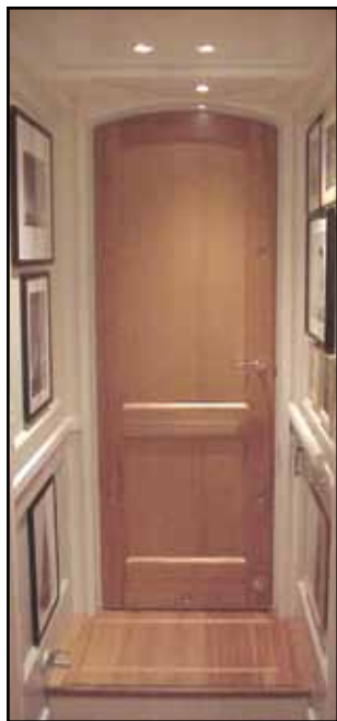
Hallway door, Mitered corners, Custom top arch, Veneered
