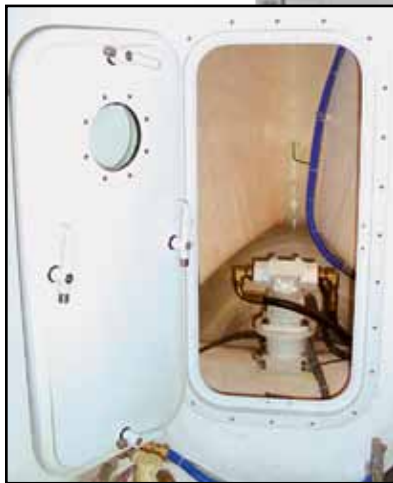
7" view port, Access to bow thruster
